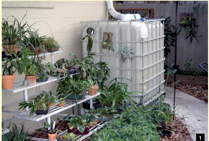
[1] Rainwater collection tank ties into roof downspout.
